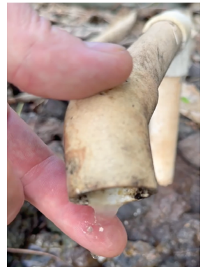
HVAC condensate completely laden with Zoogloea
